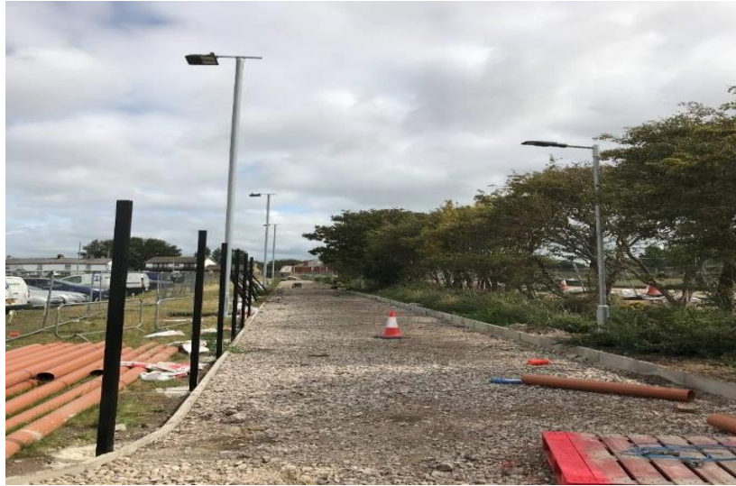
Image 9 New footpath / cycleway at Division Lane West (under construction)
